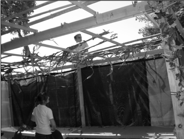
The building of the Sukkah at the AJCC.
